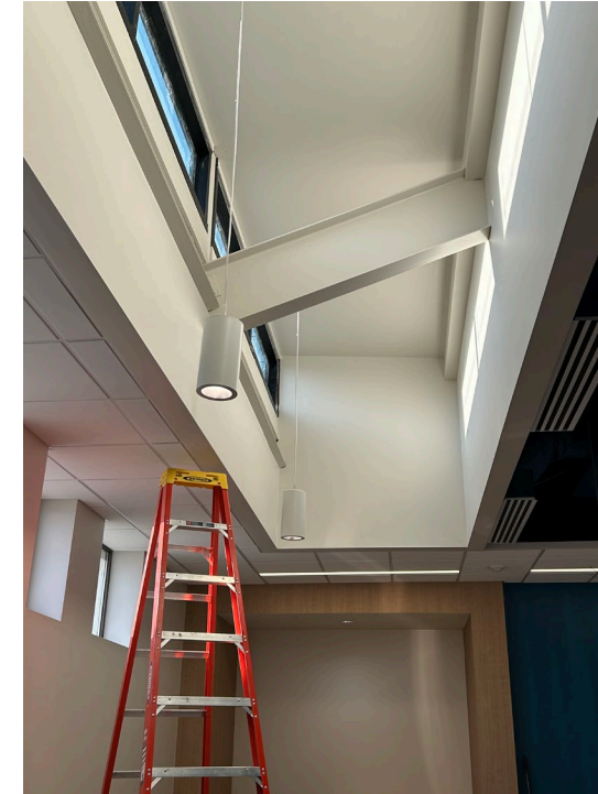
Dormer windows in the adult area. Increases ceiling height and bring in natural light
