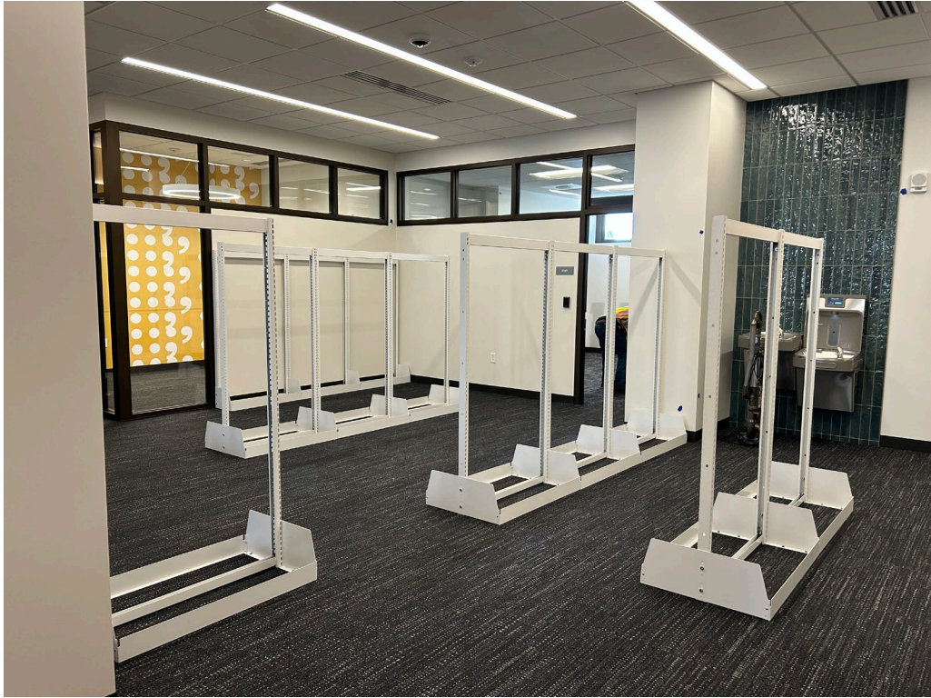
Shelving installation in progress
