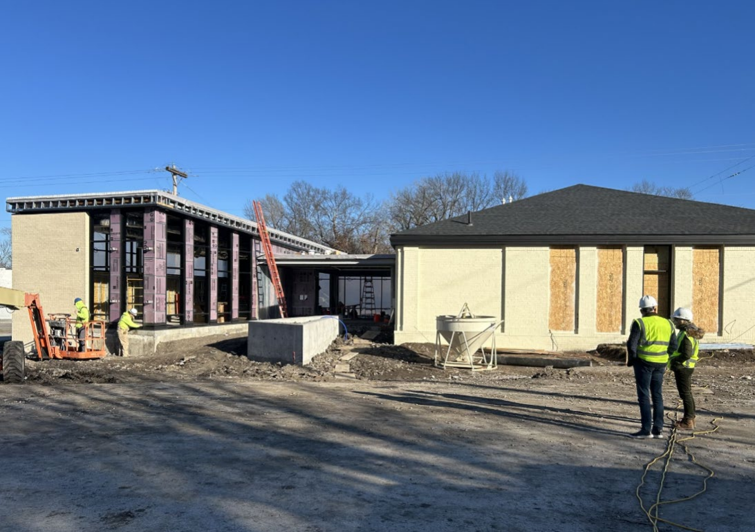
View of both structures, the original brick has been painted to compliment the new brick; new roof was installed on the original building
