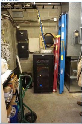
The photos here show some of the challenges of IT spaces in the library system, including incompatible use of IT space with other functions (such as power transformers, HVAC, and storage). The library has done a good job of mitigating issues (the enclosed rack in these areas is an excellent response).
