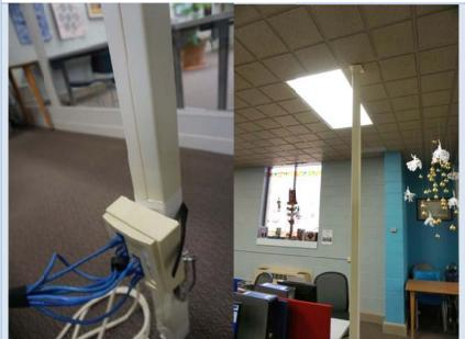
The library did an excellent job retrofitting this branch for adequate data and power by using ceiling poles and external raceways. Recommendation: all new facilities should be designed for technology flexibility over time. When possible, raised floor (also called access flooring), perhaps combined with building HVAC needs, should be specified for public areas. Raised floor allows power and data to be moved as needed to support the library's evolving service model over time.
