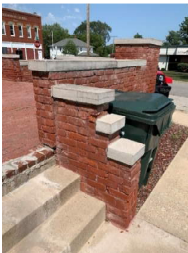
Figure 8. Spalling at Stair Wall
