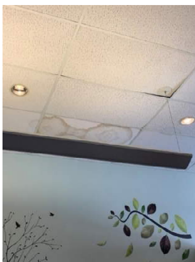
Figure 25. Water Damage on Ceiling Tiles
