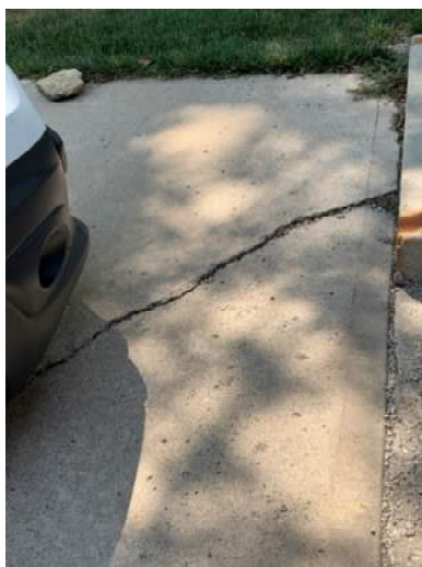
Figure 21. Cracked Sidewalk at SW Entrance
