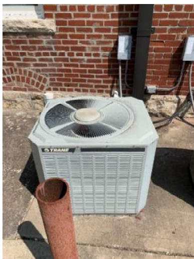
Figure 23. Condensing Unit at South Facade
