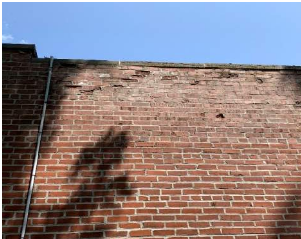
Figure 4. Brick Spalling on West Facade
