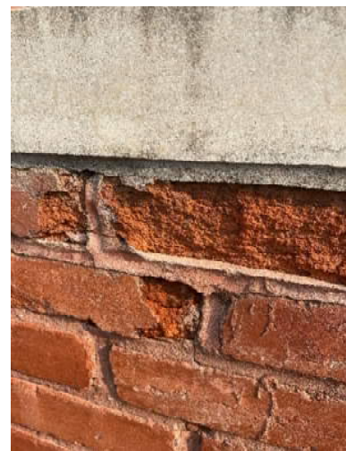
Figure 10. Spalling at Stair Wall
