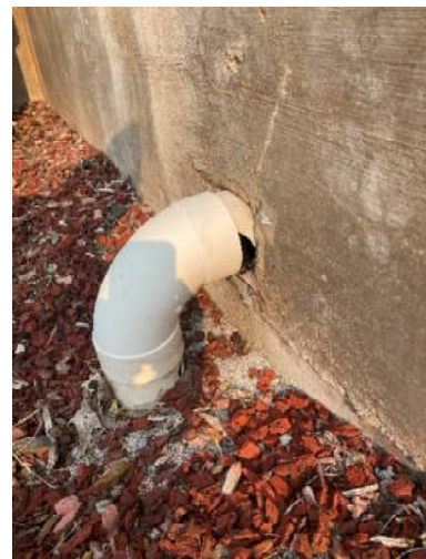
Figure 18. Cracked Drainage Pipe
