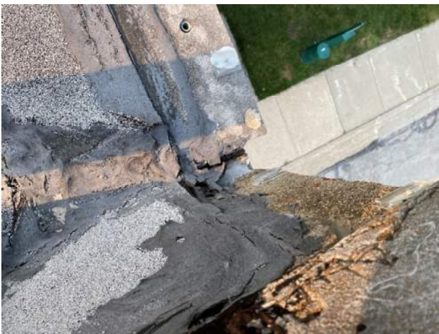
Figure 11. Roofing Gap at Building Corner
