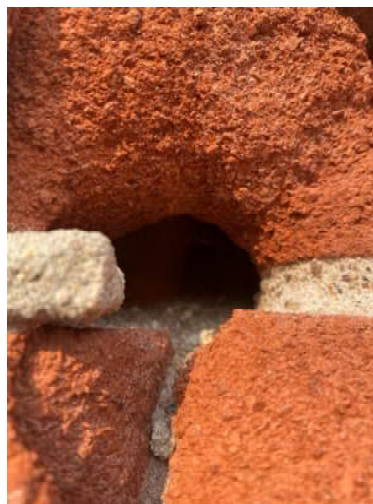
Figure 9. Grout Decay at West Patio
