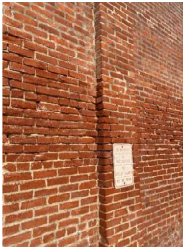
Figure 6. Grout Decay at West Patio
