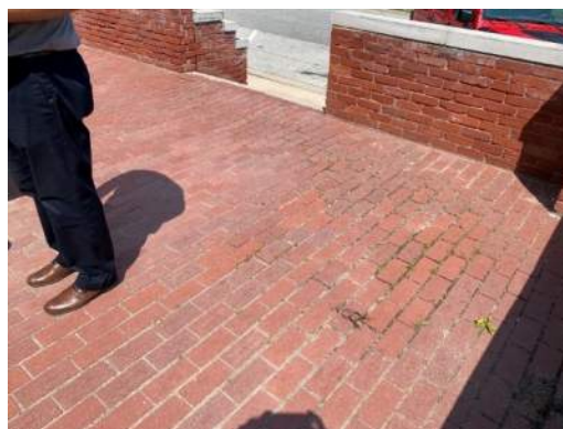
Figure 20. Sloping Patio Surface
