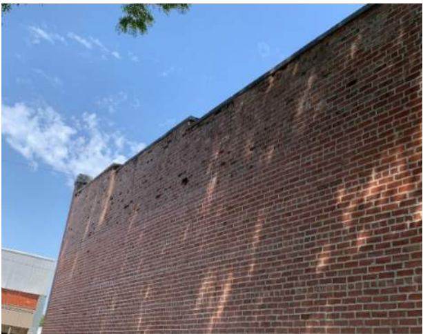
Figure 3. Brick Spalling on West Facade
