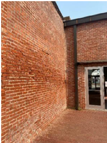
Figure 5. Grout Decay at West Patio
