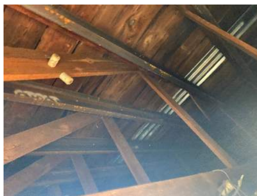
Figure 24. Rust on Steel Roof Supports
