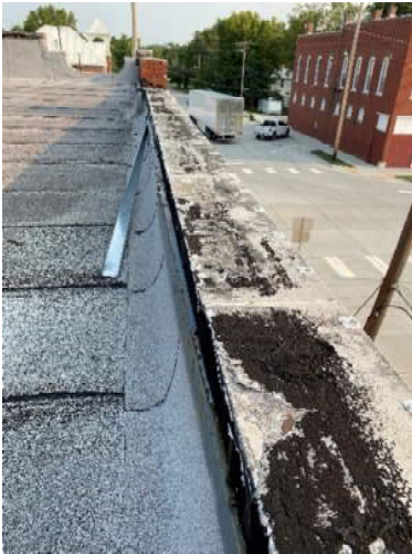
Figure 13. Torn Flashing at East Edge
