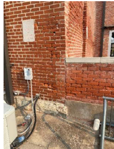
Figure 7. Grout Decay at South Wall
