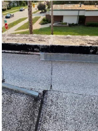
Figure 14. Torn Flashing at East Edge
